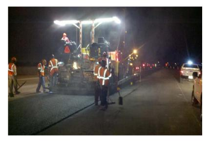
Milling consists of removing the surface of the road in preparation for new asphalt. This operation is performed with specialized milling machines, and can generate noise. FDOT will be monitoring decibel levels to ensure that the contractor stays within tolerance. Paving requires the use of a vibratory roller to ensure proper compaction of asphalt; vibration monitors will be in place for the duration of this activity and will be monitored and reviewed by FDOT staff.
