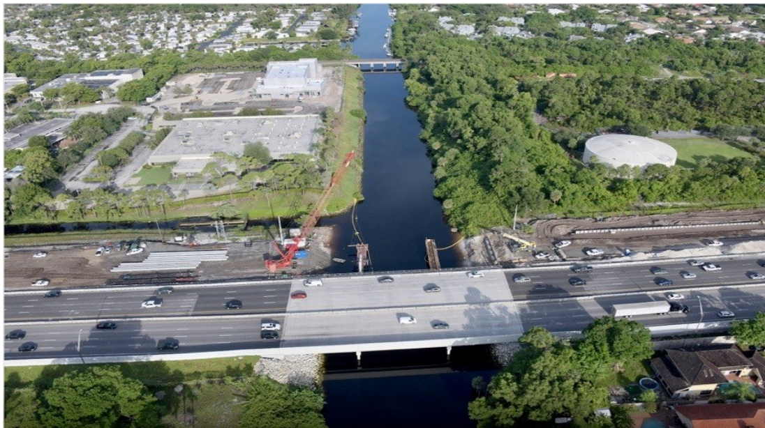
Aerial View of I-95 southbound widening at Hillsboro Canal
