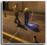
Loop installation consisting of vehicle detection system cut into asphalt at the beginning of the entrance ramp as well as at the Ramp Signal location
