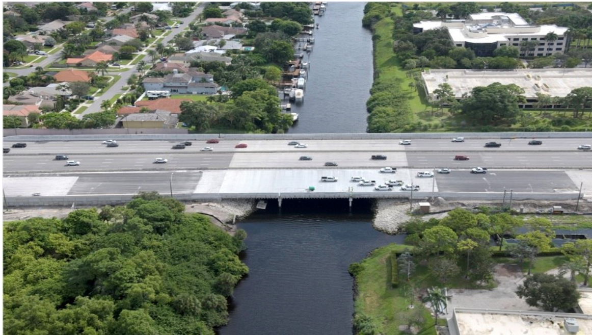
aerial view of the newly reconstructed Hillsboro Canal Bridge looking east
